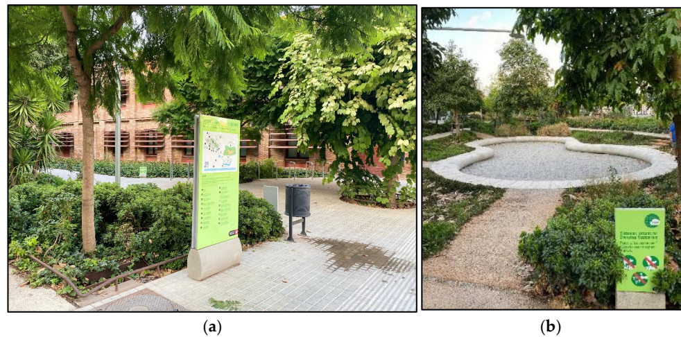
Figure 7. Sustainable Urban Drainage System (SUDS) in Barcelona (a,b). Source: author (2024).
