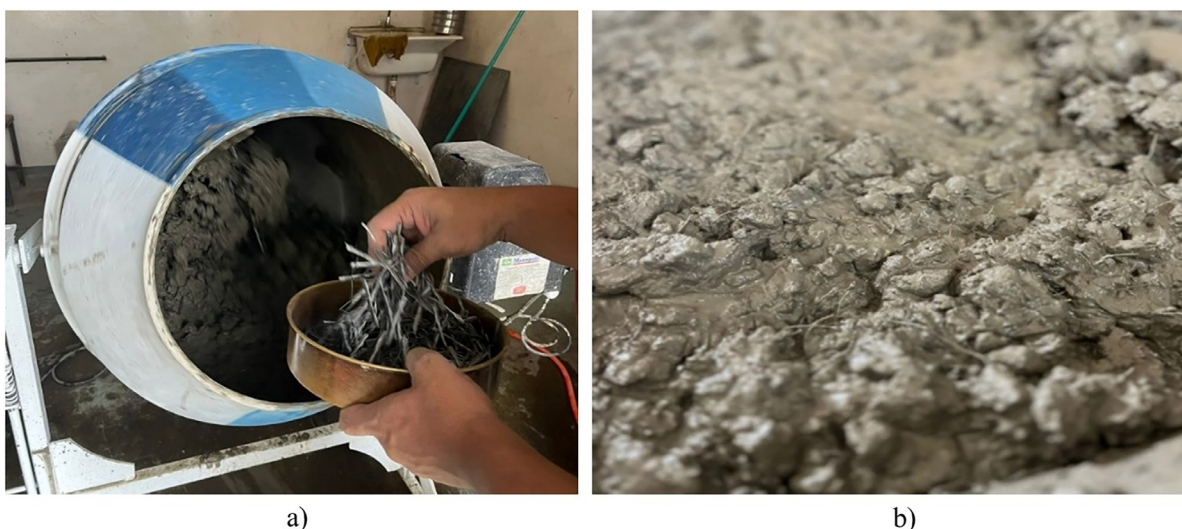
Figure 3: The addition of fiber into the concrete (left) and concrete in the fresh state (right).
