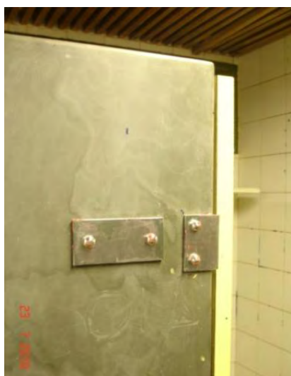
Figura 4.52 - Ferragens fixando as pedras de boxes
