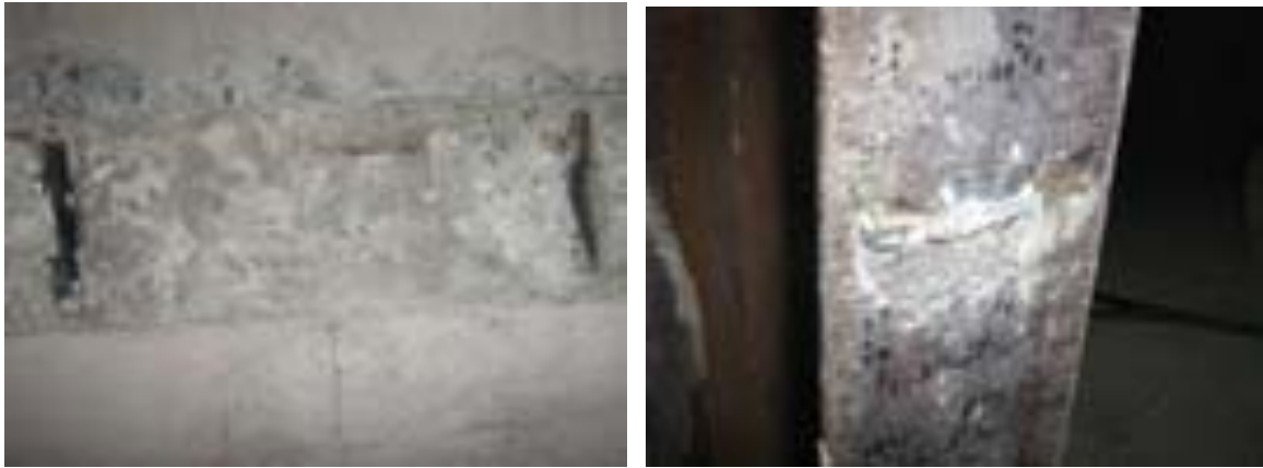
(a) Ruptura do conector
